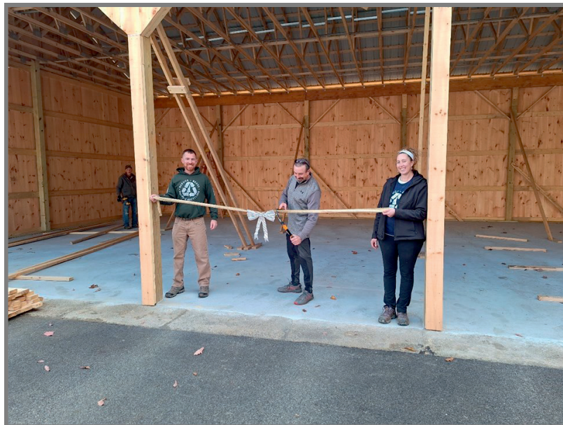
Pole Barn at the Recycling Center Completed in November 2023
