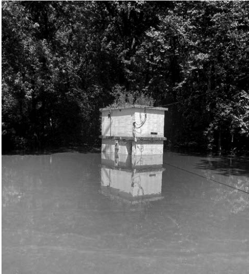
Flooding at River Well July 11, 2023 (File photo)
