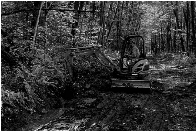
Ditch work on the rail trail by SnowHawk LLC
